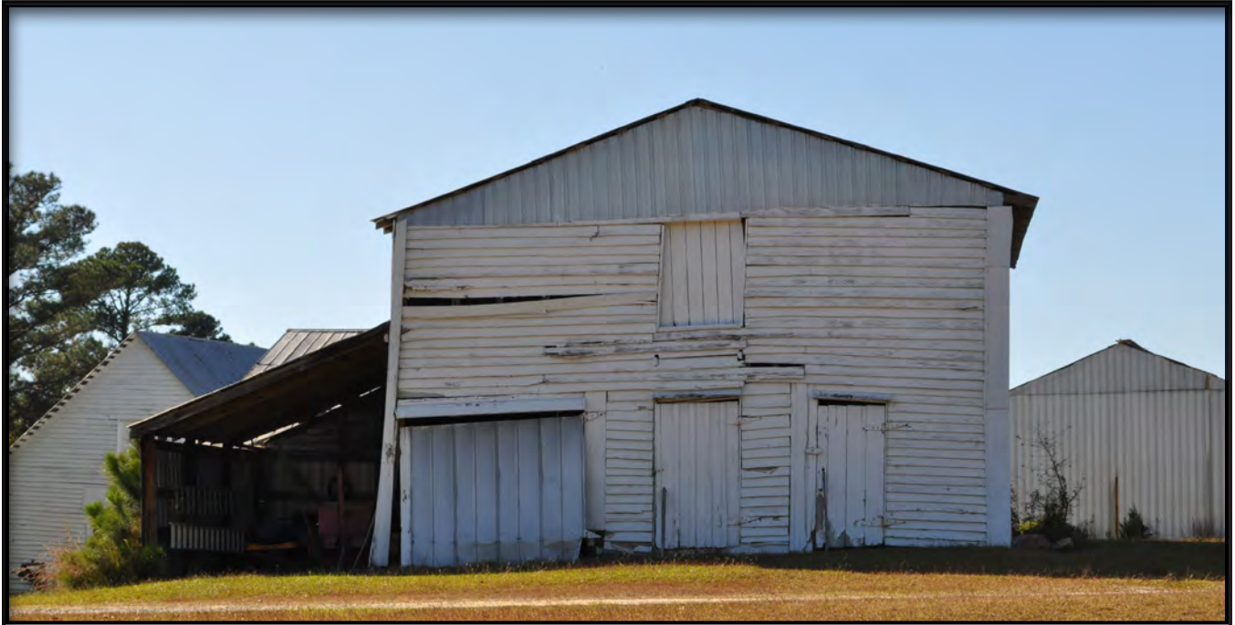
Figure 24. Livestock Barn #1, East Elevation
