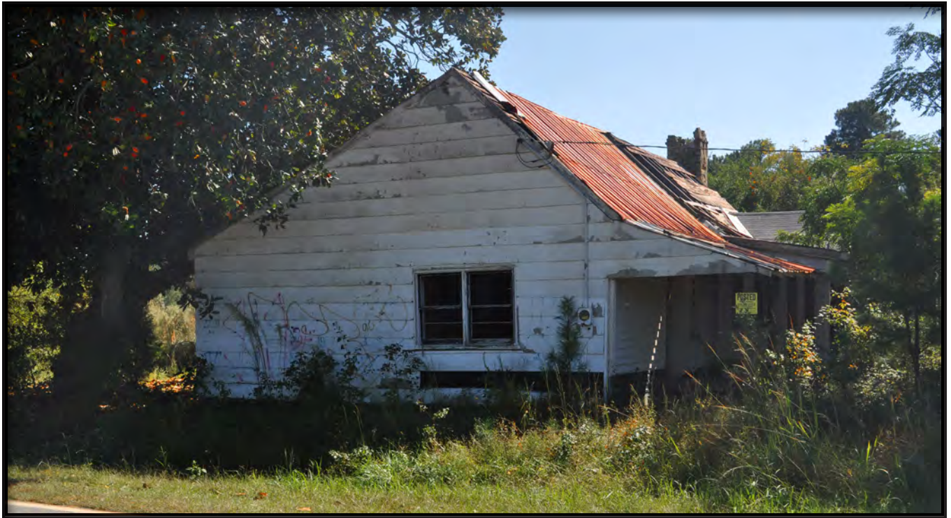
Figure 32. East Elevation, Looking Southwest from Pierce Road
