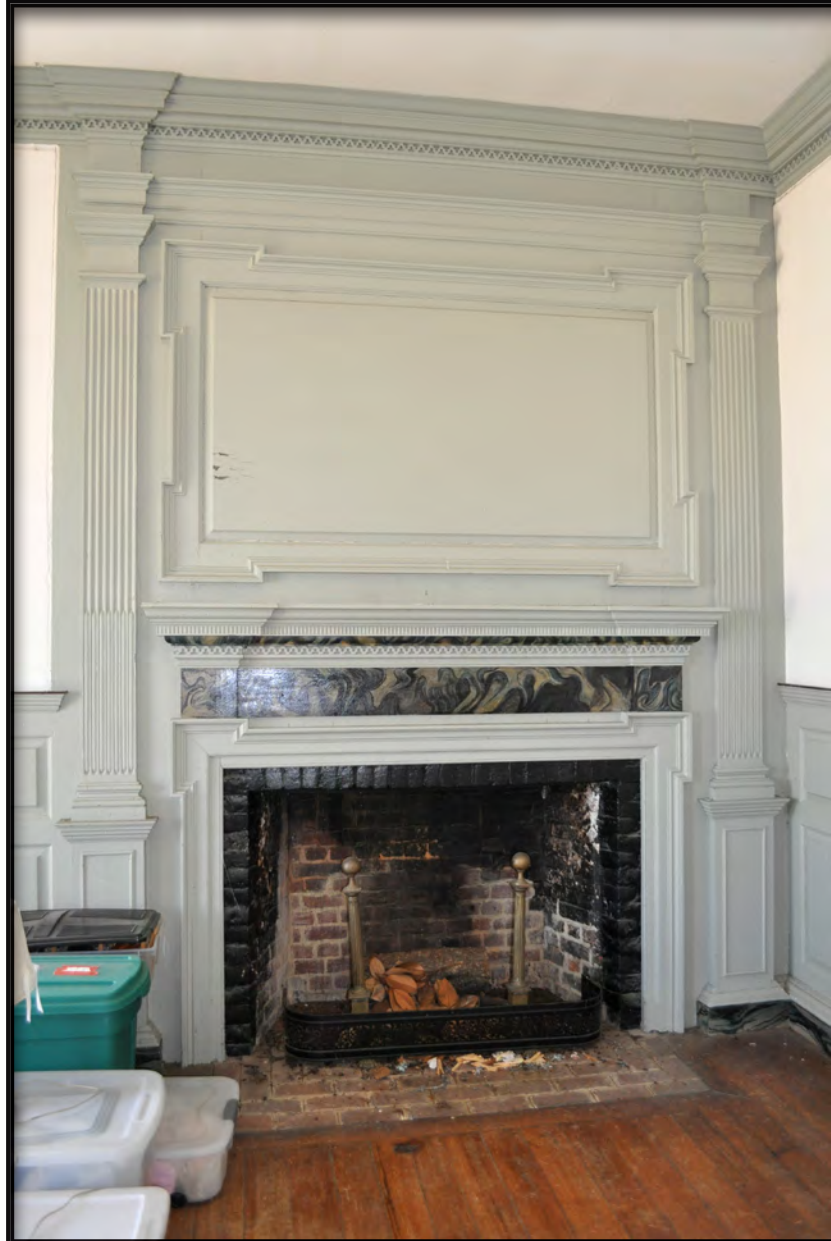
Figure 9. View of Hall Fireplace Showing Mantel and Overmantel with Original Marbled Paint
