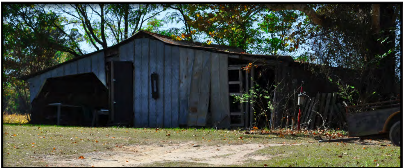
Figure 53. East Side of Shed
