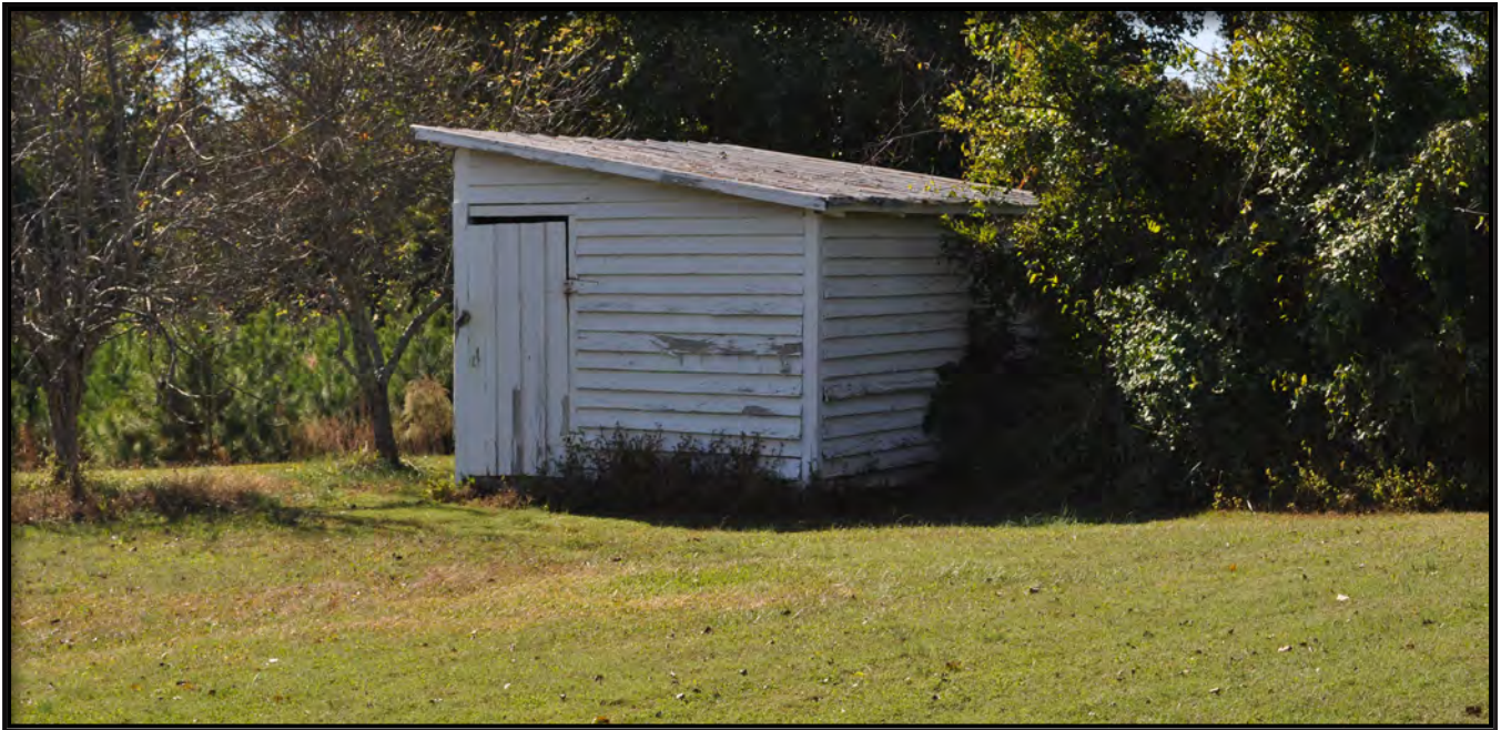
Figure 23. East Elevation of Garden Shed
