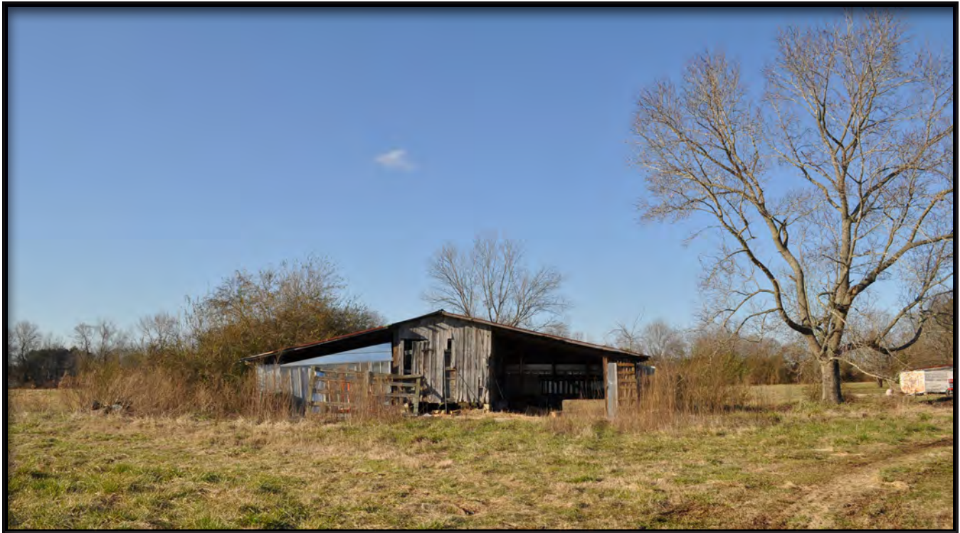
Figure 12. Barn 1, South Side
