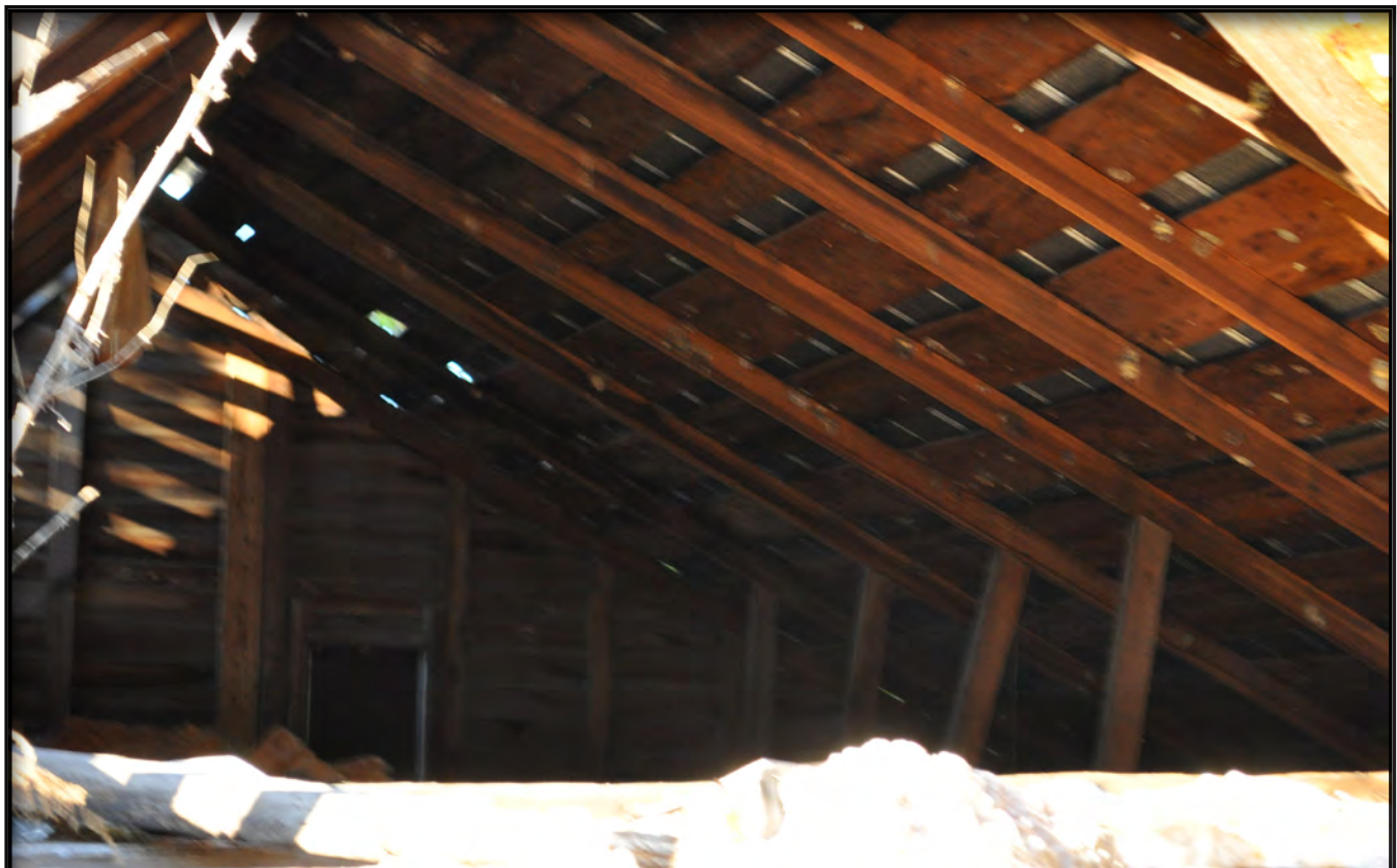
Figure 42. View of Rafters and Skip Sheathing in of Mid-Nineteenth-Century Addition
