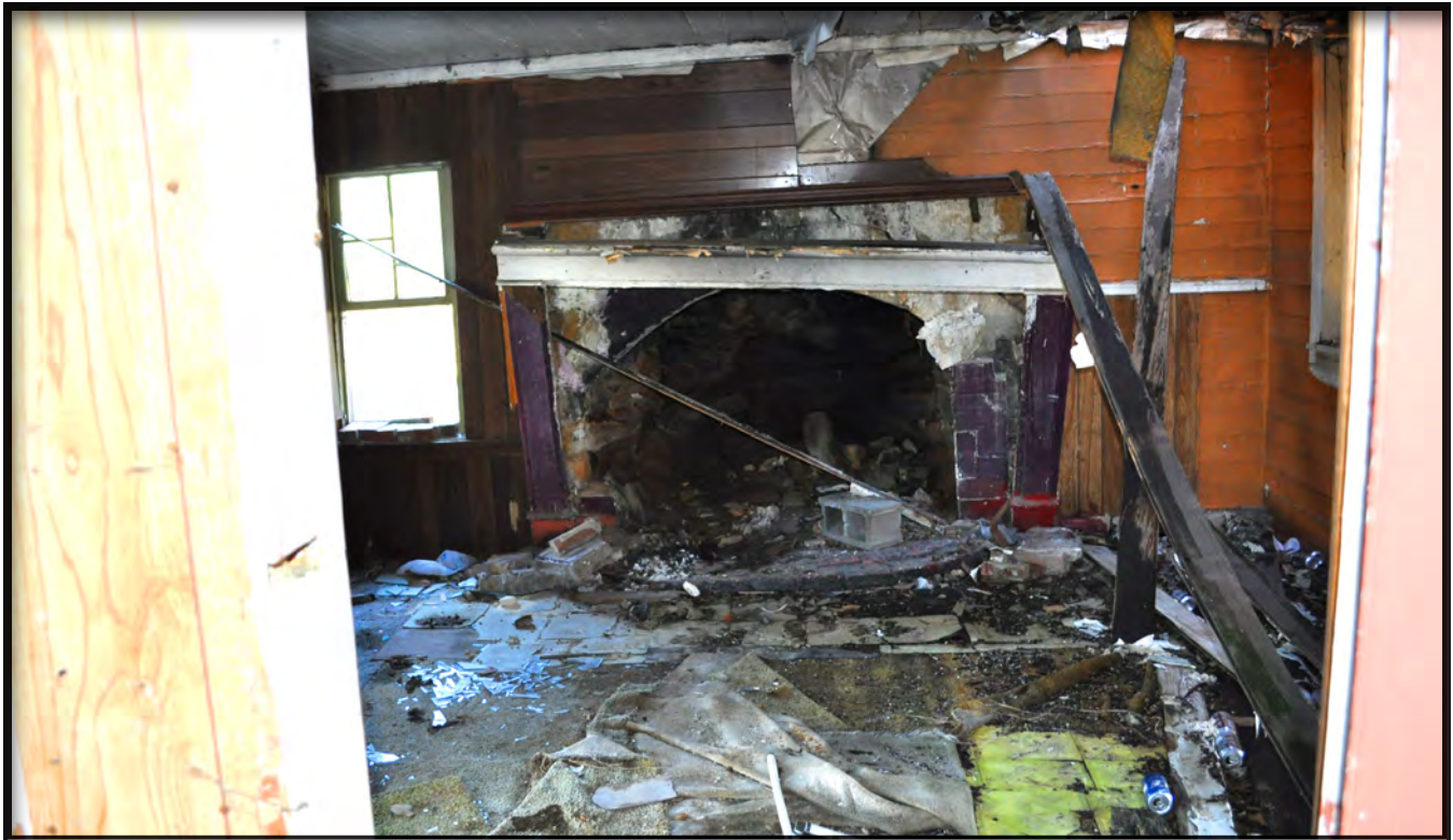
Figure 44. View from South Room Looking South to Firebox and Mantel
