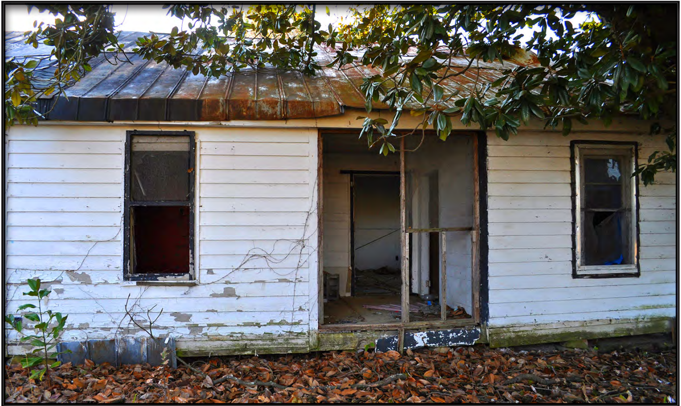
Figure 34. East Elevation Showing Mid-Nineteenth-Century Addition with Shed Rooms
