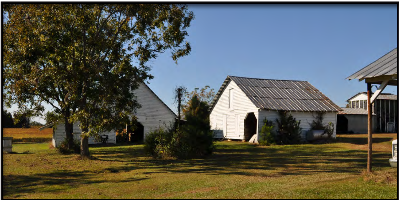
Figure 25. Livestock Barns #2 and #3, Taken from Carport Looking Northwest
