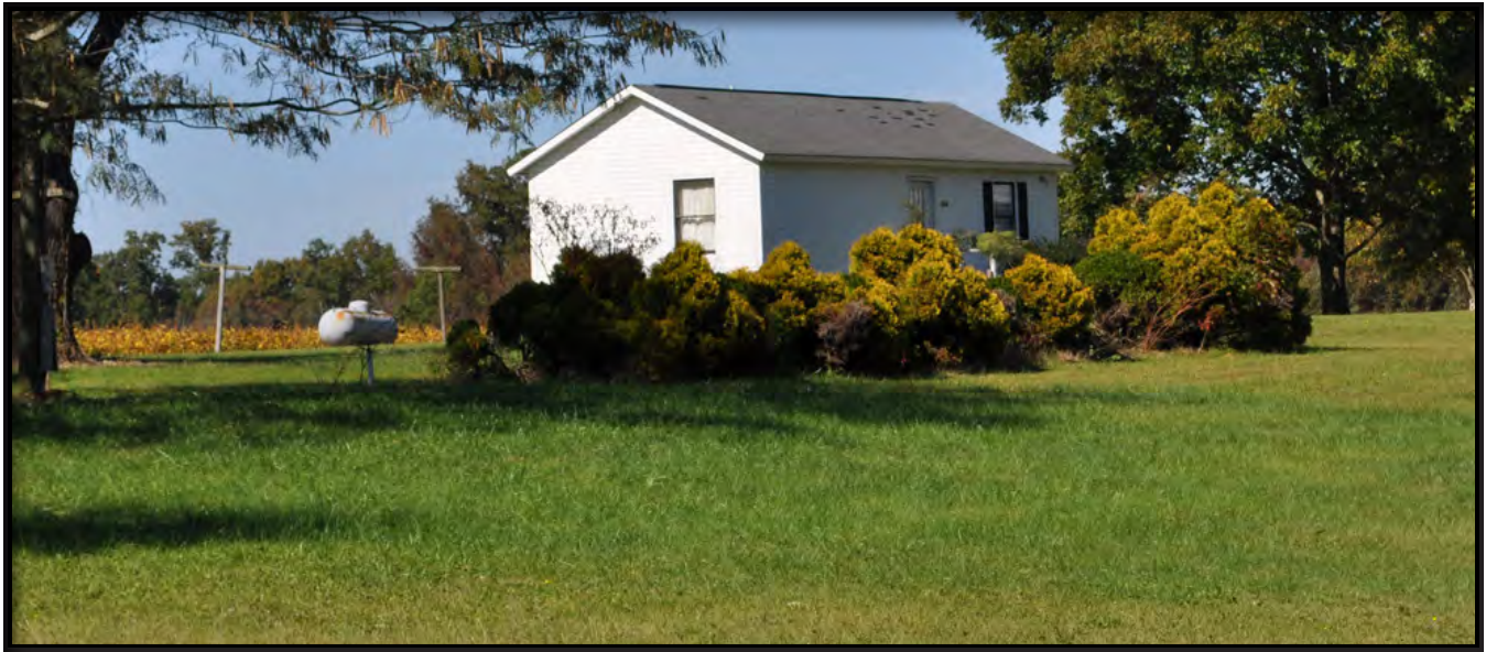
Figure 49. Front (East) Elevation of Modern Dwelling South of House
