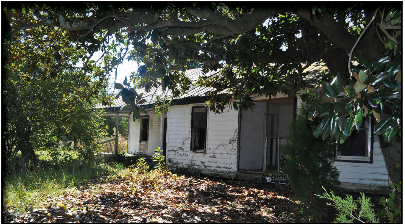
Figure 33. North Elevation Showing circa 1830s Section
