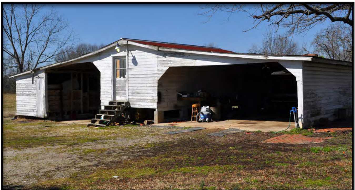
Figure 11. Tractor/Car Garage and Workshop, South Side
