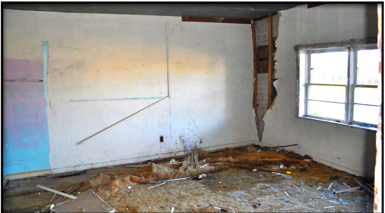
Figure 40. View of North Room Looking Northwest
