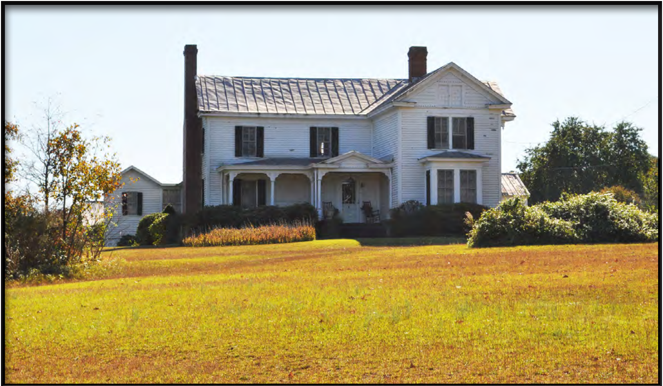
Figure 17. Front (North) Elevation, Note Original Kitchen Left of Frame
