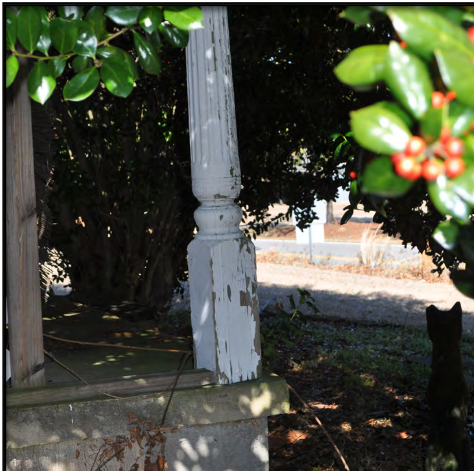
Figure 51. Detail of Porch Post on Front (East) Porch
