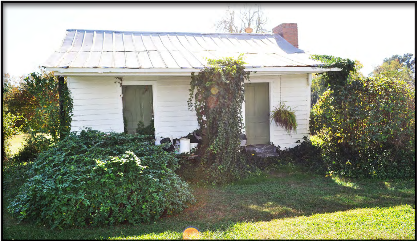
Figure 21. North Elevation of Laundry/Kitchen
