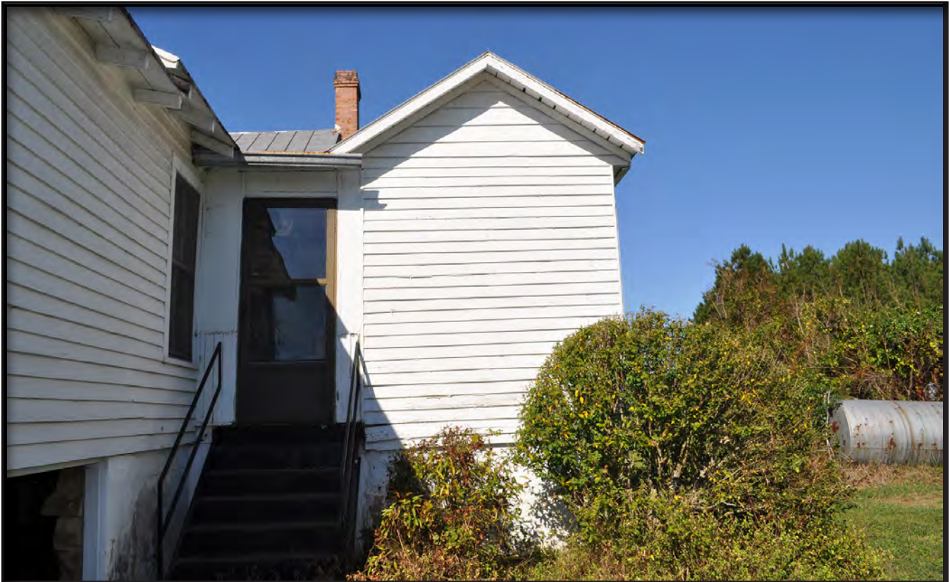
Figure 19. Rear (South) Elevation of Original Dairy with Connector on East Side of Main Dwelling
