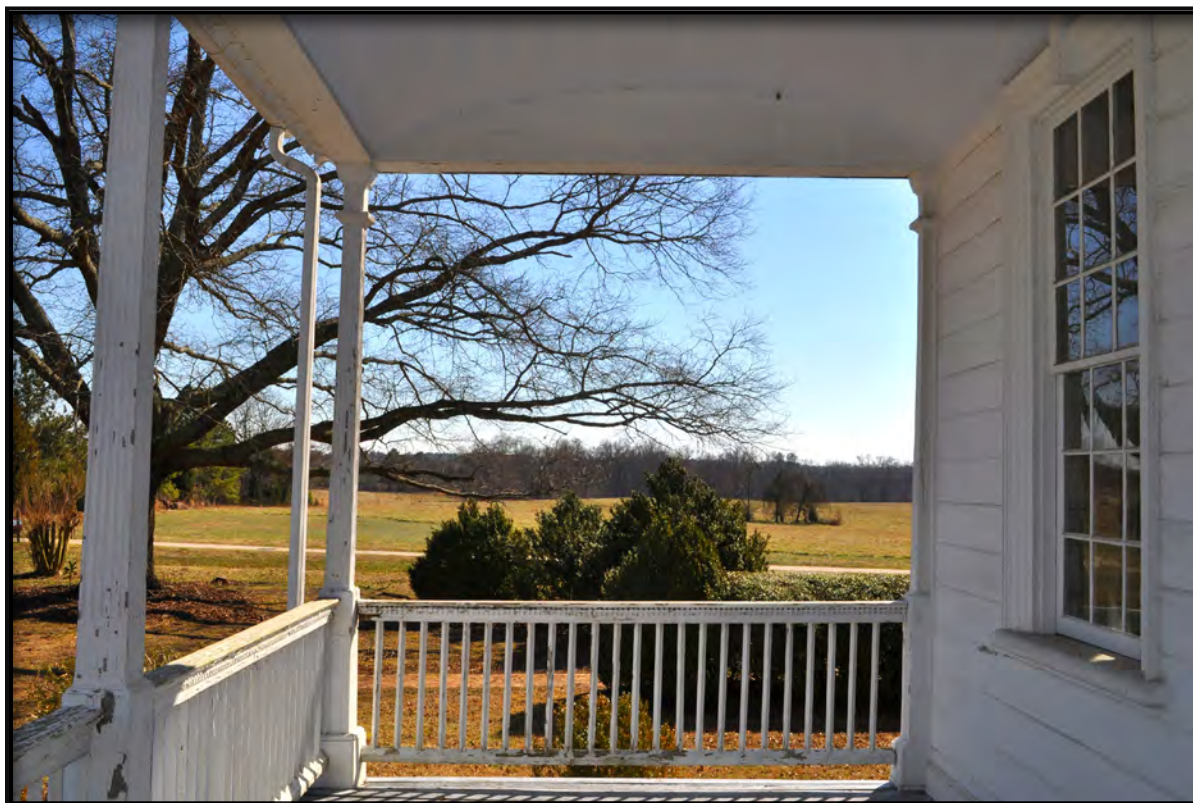
Figure 6. Porch Vaulted Ceiling, "Keystone" Window Surround, Fluted Columns and Balustrade with Dentilated Handrail, Looking South with Fields in Background
