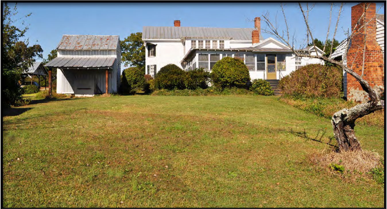
Figure 18. North and West Elevations Showing Enclosed Sun Porch at Rear of Dwelling, Smokehouse Right of Frame
