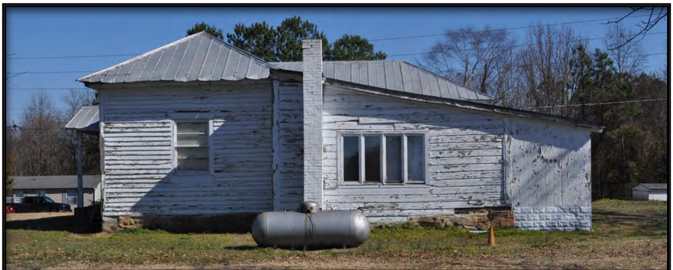
Figure 54. West (Rear) Elevation
